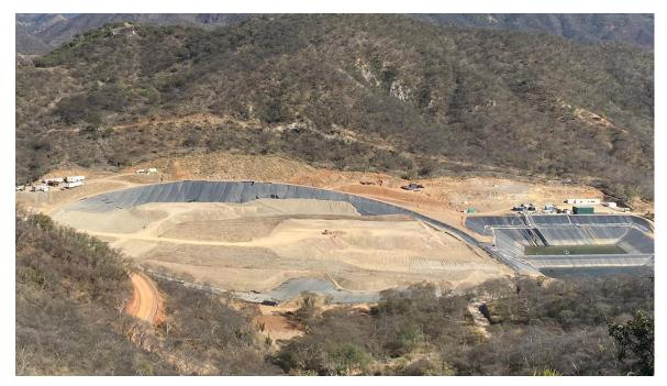
Photo 1: Advancement of stacking and leaching activities at Santana heap leach pad
