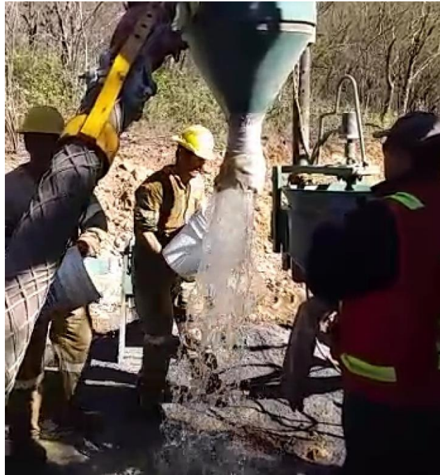
Photo 1 – Successful Water flow identified in WDH4
